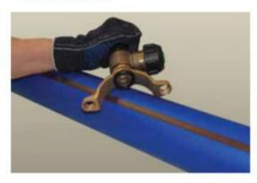
Fit the self-tapping ferrule squarely around the main and tighten the two strap bolts evenly and symmetrically.
