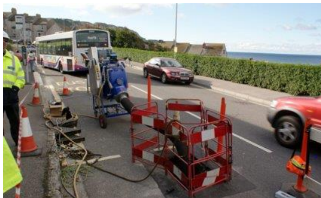
Fig 2: Aqualiner inversion bag to drive pig
